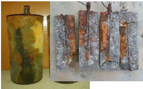
Figure.3. Corroded Bars, Cleaning of Bars with Chemical Solution
