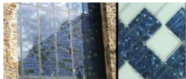
Fig. 4. PV cells as element of building patterns [38]
