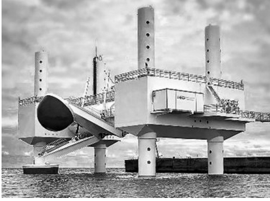
Figure 3: Wavestar prototype at Hanstholm with one floater (left) in operational mode and the other (right) in storm protection mode.
