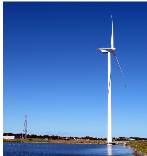
Figure 1–2 A classic three-bladed horizontal-axis Vestas V90-3.0 MW offshore wind turbine installed on a bucket foundation.
