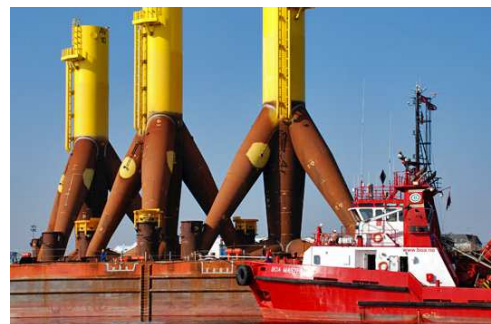
Figure 1–9 Tripod foundations for the Alpha Ventus offshore wind farm with a pre-installed pile method. (Geniusstrande 2014)
