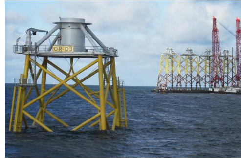
Figure 1–10 Jacket foundations for the Ormonde offshore wind farm. (Peire et al. 2008b)
